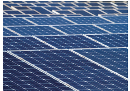
Solar Array Load Testing
