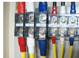
Locations with covered terminals
